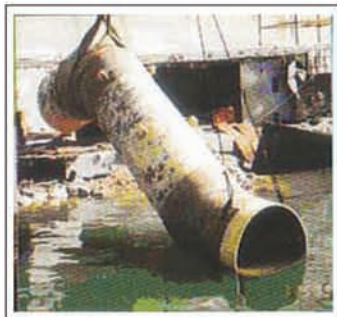
Underwater Pipeline Works
