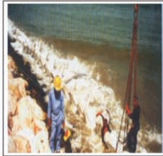
Underwater Core Lock Fixing & Rock Foundation Core Rock Filling
