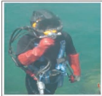
Sea Water intake Pipe Line Works
